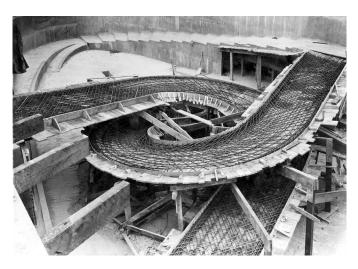
Figure 2: Reinforced concrete in the construction of the penguin pool at London Zoo.
